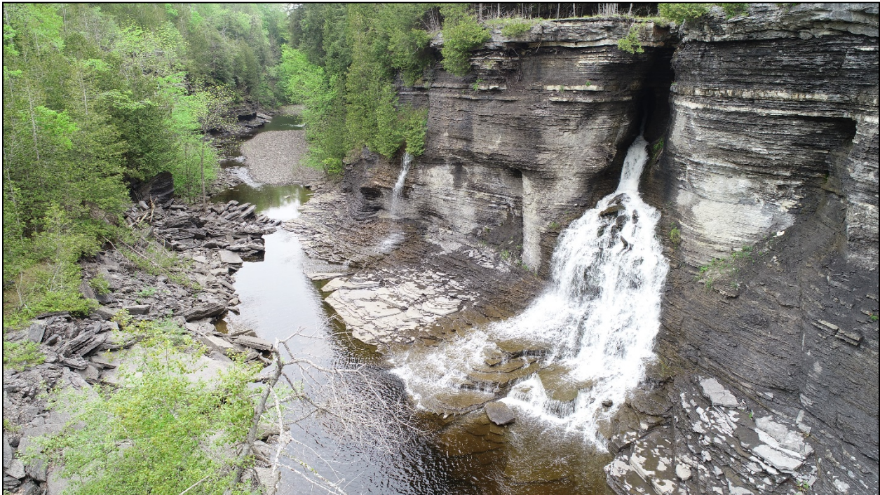
PHOTO D-4 LOOKING UPSTREAM TO JUST BELOW MILITARY BRIDGE AREA
