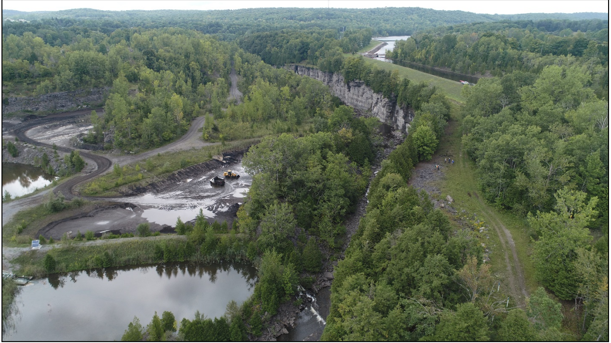
PHOTO D-9 LOOKING UPSTREAM TO POWER CANAL
