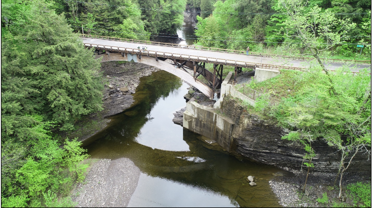
PHOTO D-1 LOOKING UPSTREAM TO MILITARY BRIDGE AREA
