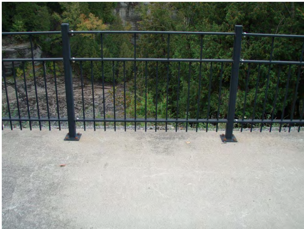
Photo 1. Trenton Trails Accessible Overlook Railing – 24 Sep 2019
