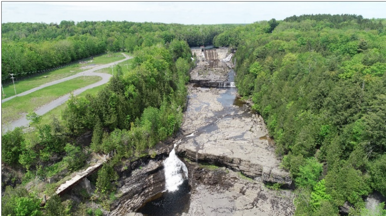
Photo 3-4 Upper Portion of Trenton Bypass Reach
