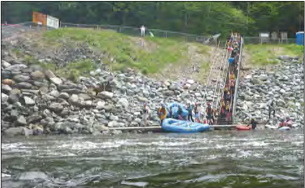
Photo 12: Deerfield No.5 river access (MA) constructed by the FERC licensee to provide river access in an area with steep banks. A similar solution may be used to provide access to the Trenton impoundment.
