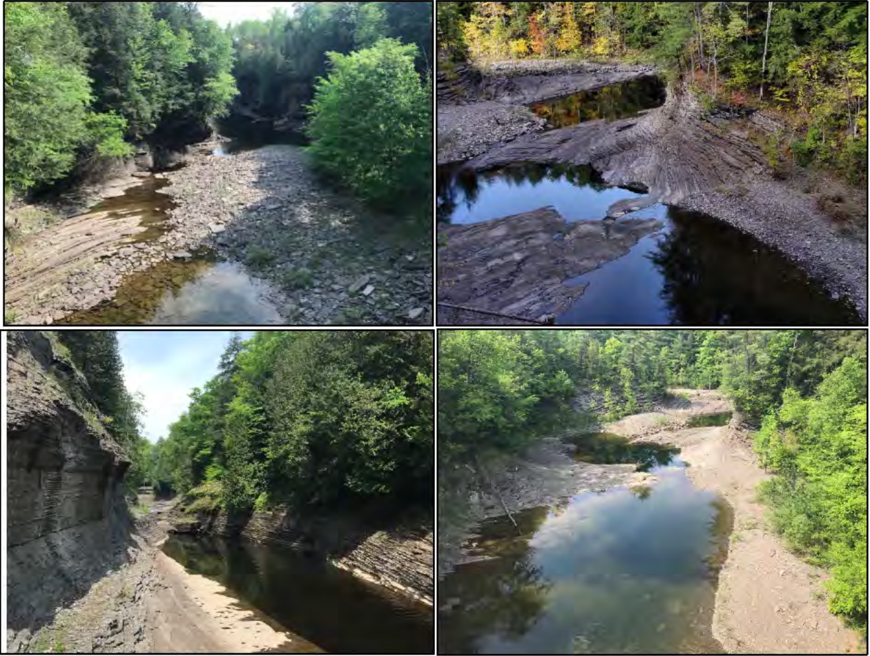
Photo 2: Prospect bypass reach dewatered.
