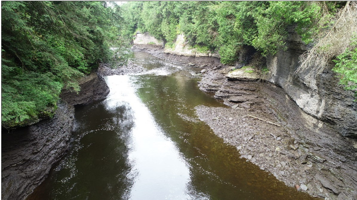
Photo 3-3 Trenton Impoundment Boulder and Cobble Deposits
